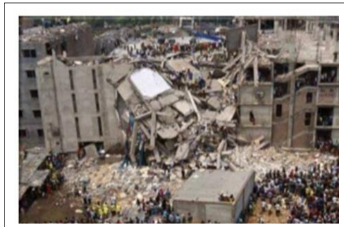
Figure 1b: Aerial View of Collapsed Structure (Source: Oke et al 2024; Akinyemi et al 2019)
