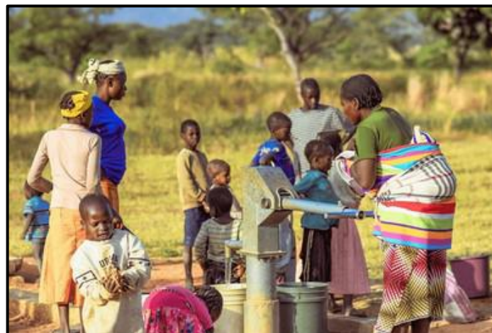
Figure 14: Hand operated borehole for safe drinking water
