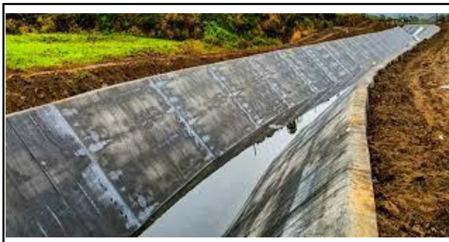
Figure 11: Concreting of irrigation canal for snail control
