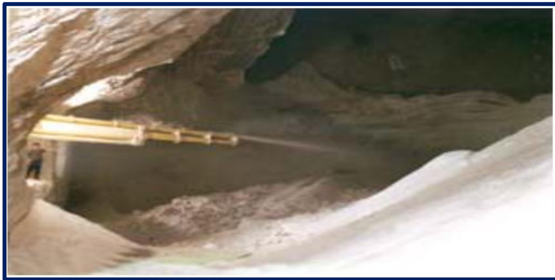
Fig 4: Backfilling a chamber at the 637-level former potash mine Ronnenberg, Germany (Helmholtz Zentrum München, 2010)
